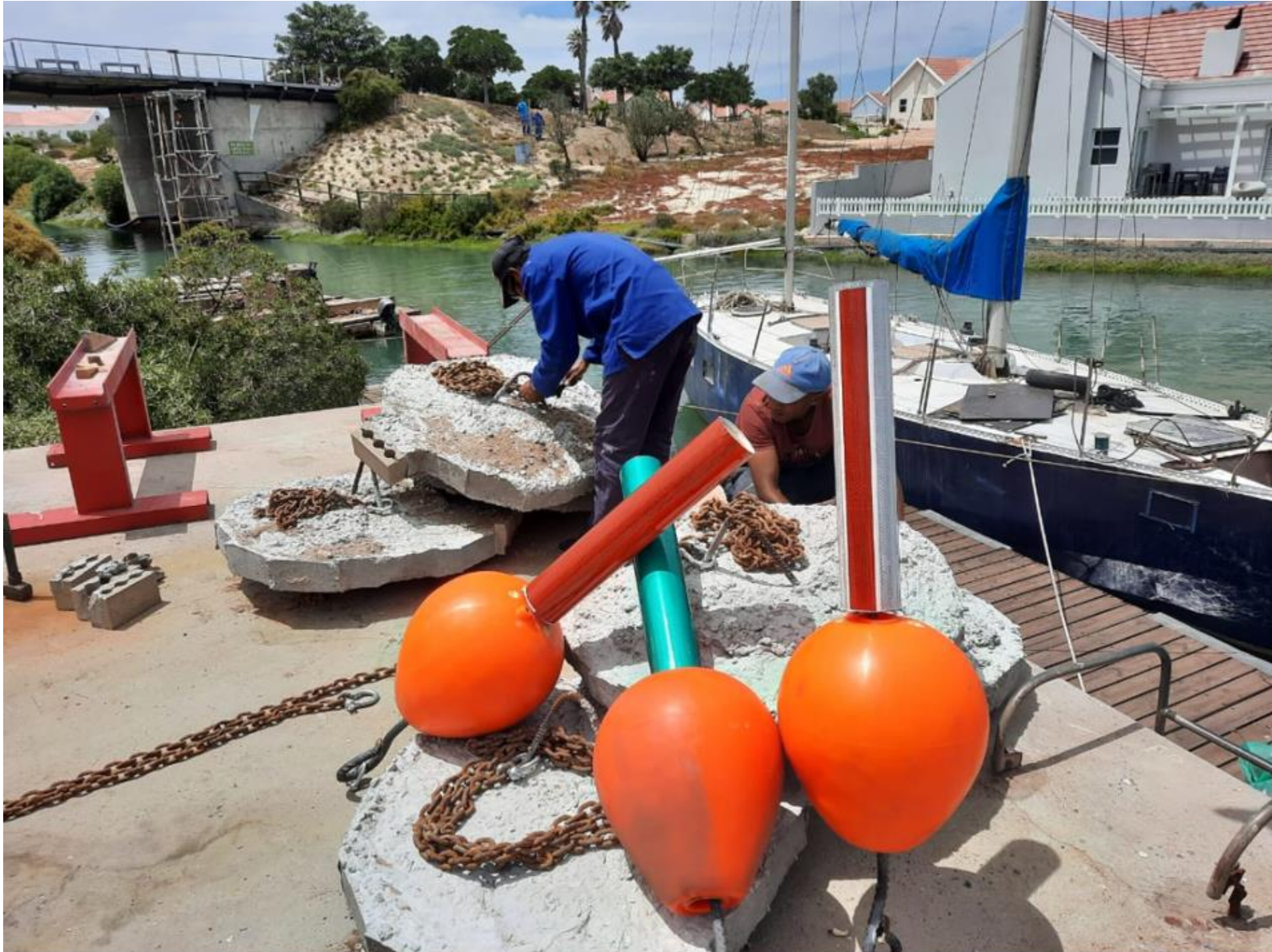
Temporary buoys and moorings being assembled
