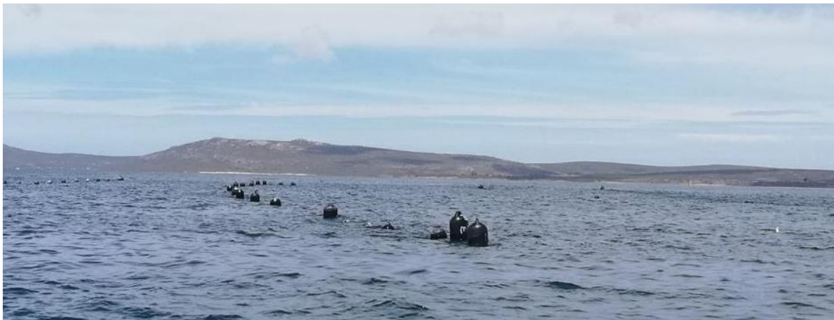
Figure 12. Mika line 3 bowed and slack indicating that the mooring has shifted and needs to be moved back to its original position.
