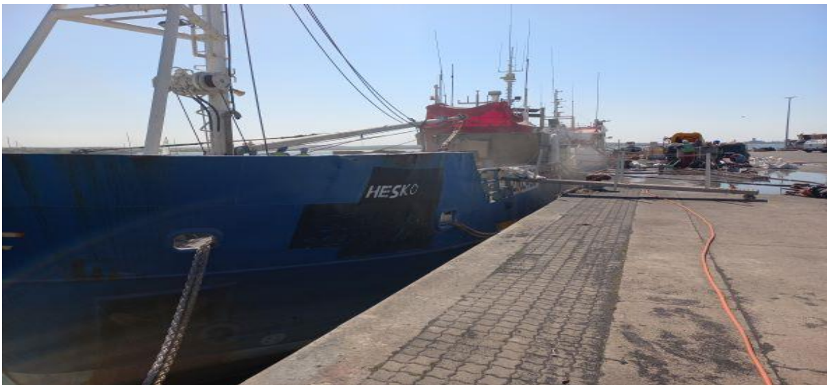
Picture 5 : Refurbishments currently being conducted.
