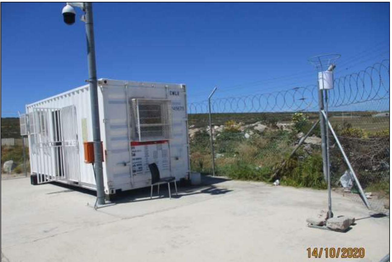
Photograph 3: Full extent of infrastructure within the mining right area.
