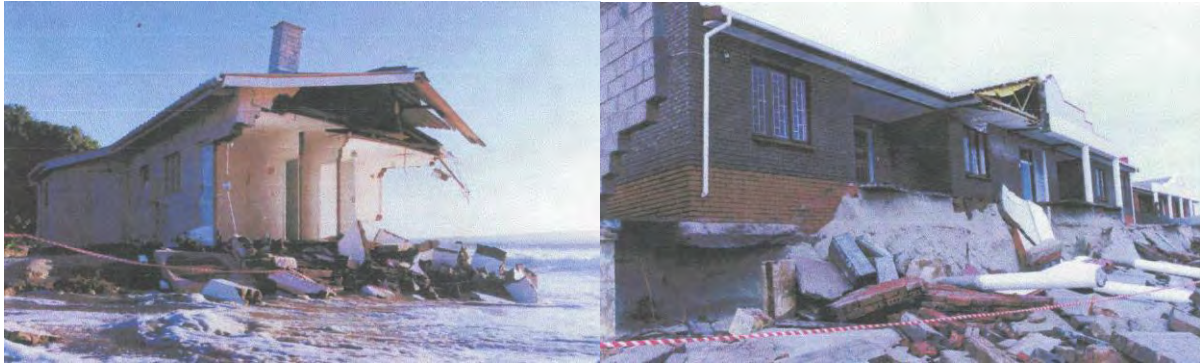
Figure 7.6. Damage to houses in Langebaan caused by a severe storm in June 1997.
