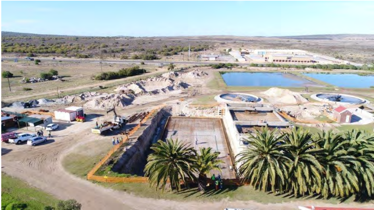
Figure 3.28. Construction activities for the upgrade of the Langebaan Waste Water Treatment Plant to increase treatment capacity and improve treatment processes (Source: Saldanha Bay Municipality).
