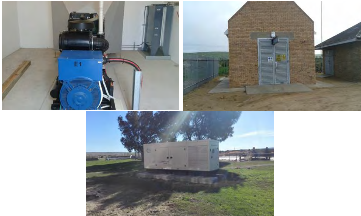
Figure 3.19. Emergency generators that have been installed at various pump stations in Saldanha Bay and Langebaan Lagoon (Source: SBM, Gavin Williams, 2016).
