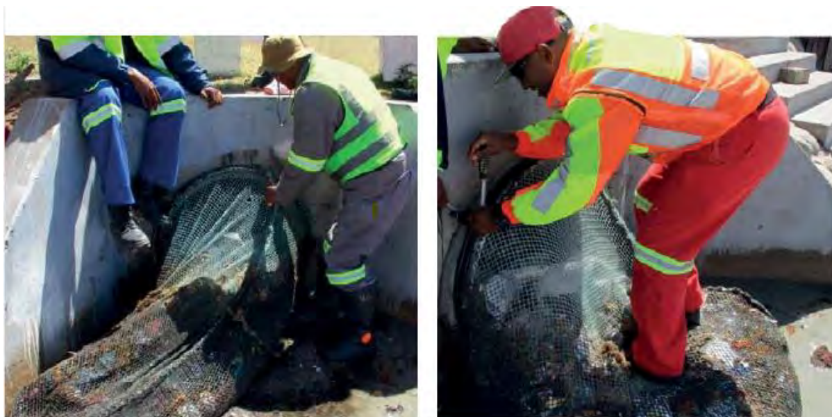
Figure 3.43. A stormwater litter trap installed in Saldanha Bay to prevent litter entering the Bay (Source: SADSTIA annual report 2019).
