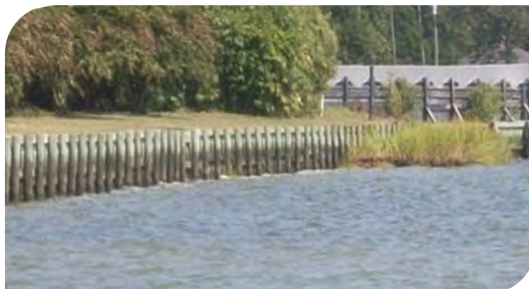
Figure 8: Example of a post-supported wall (VIMS, 2019)
