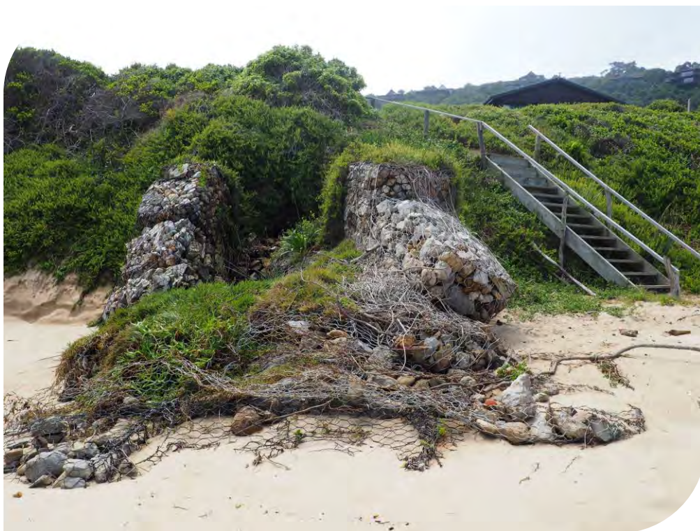
Figure 9: Gabion protection for a stormwater outlet damaged by wave action
