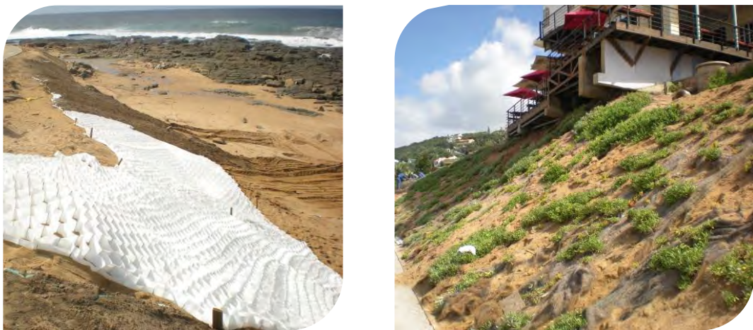
Figure 4: Example of soft stabilisation techniques which promote vegetation establishment, including honeycomb meshing (left) and hessian sheeting (right) (SSI, 2011)
