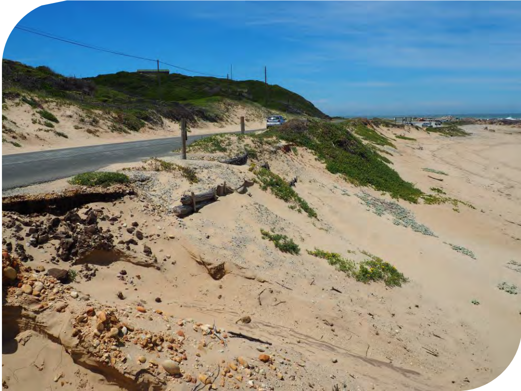
Figure 11: Wave and wind erosion on a road, Goukamma
