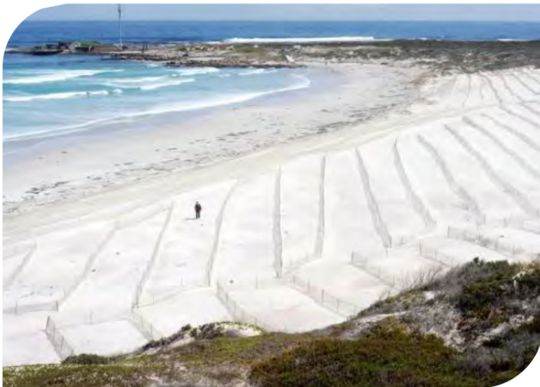
Figure 2: Entrapment of wind-blown sand using netting, Witsands Beach (Bamford, 2016)
