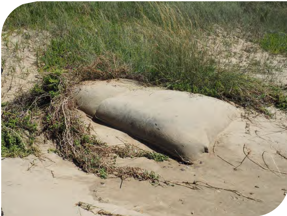
Figure 6: Sand filled geotextile bags exposed by wave action
