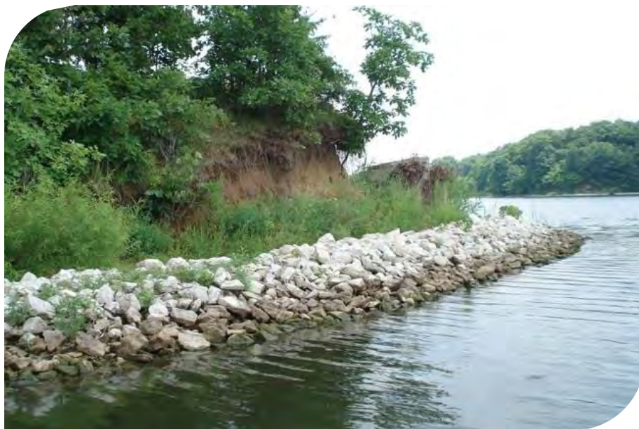
Figure 5: Example of rip-rap revetment protection (source: shorelinemetrics.com )
