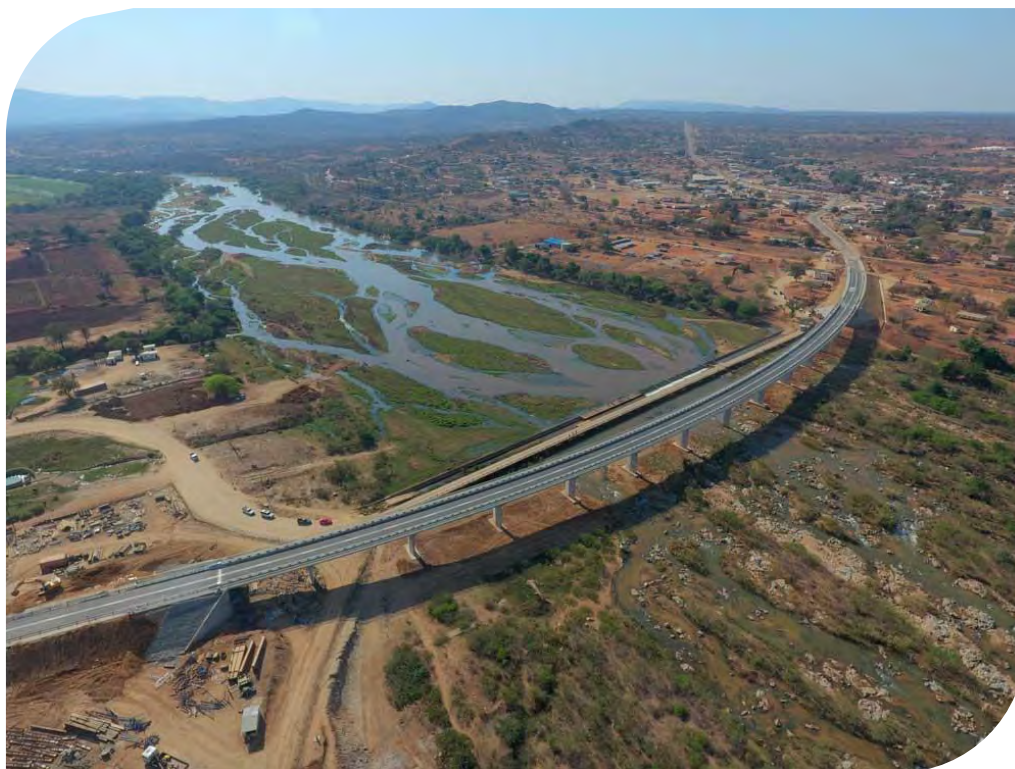
Figure 15: Siphofaneni Bridge, Eswatini, with minimal impact on the hydraulic properties of the river (Image: Aurecon)
