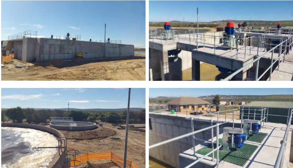
**Figure 3.22** The pictures show the new aerator basin, digester and mechanical equipment at the Saldanha Waste Water Treatment Works (Source: SBM, Gavin Williams, 2016).
