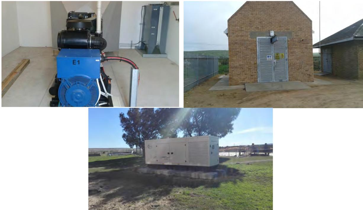
**Figure 3.20** Emergency generators that have been installed at various pump stations in Saldanha Bay and Langebaan Lagoon (Source: SBM, Gavin Williams, 2016).
