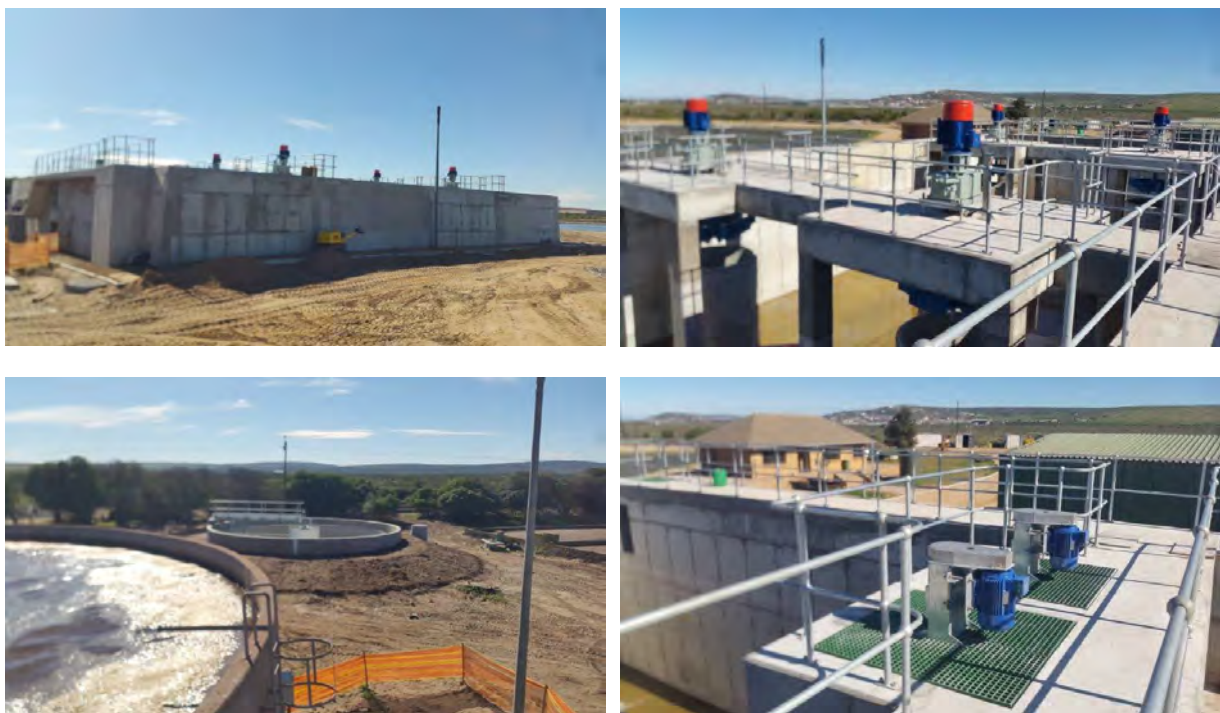
Figure 3.24 The pictures show the new aerator basin, digester and mechanical equipment at the Saldanha Waste Water Treatment Works (Source: SBM, Gavin Williams, 2016).
