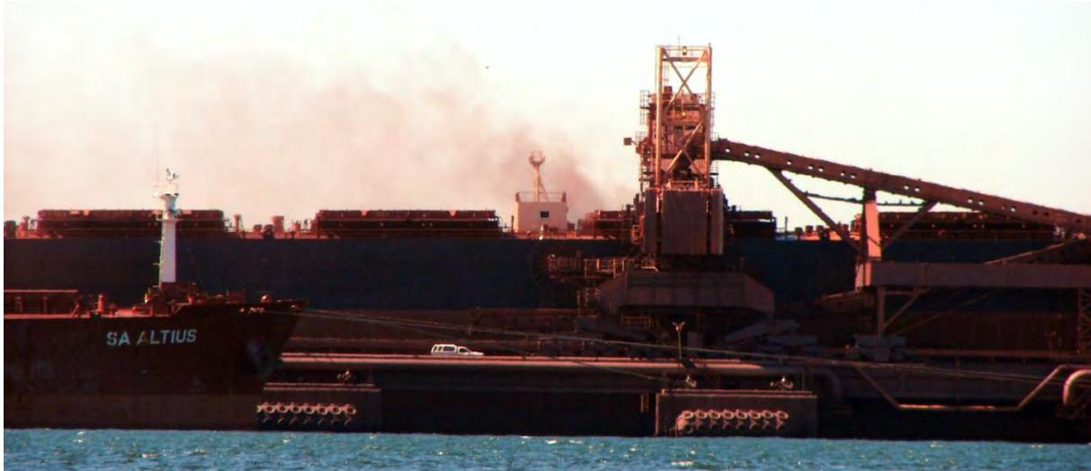
**Figure 3.16** An iron ore vessel being loaded showing associated iron ore dust emission. Freshwater from the Transnet RO plant will be used to mitigate this impact by wetting the ore before loading.
