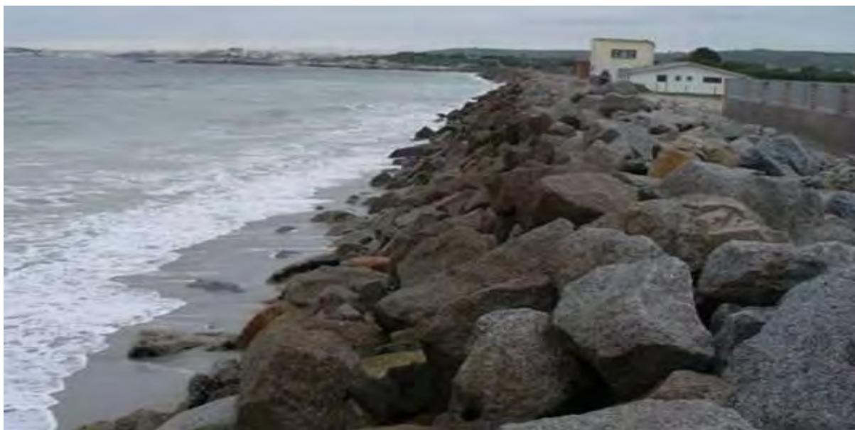
**Figure 5.5. Rock revetments constructed along the beach at Langebaan in an effort to protect coastal infrastructure.**
