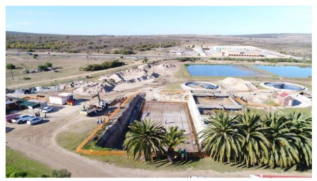
Figure 3.29 Construction activities for the upgrade of the Langebaan Waste Water Treatment Plant to increase treatment capacity and improve treatment processes.
