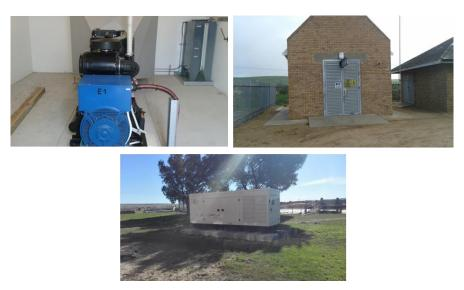
Figure 3.20 Emergency generators that have been installed at various pump stations in Saldanha Bay and Langebaan Lagoon (Source: SBM, Gavin Williams 2016).
