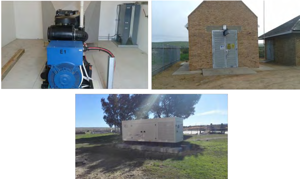
Figure 3-20 Emergency generators that have been installed at various pump stations in Saldanha Bay and Langebaan Lagoon (Source: SBM, Gavin Williams 2016).
