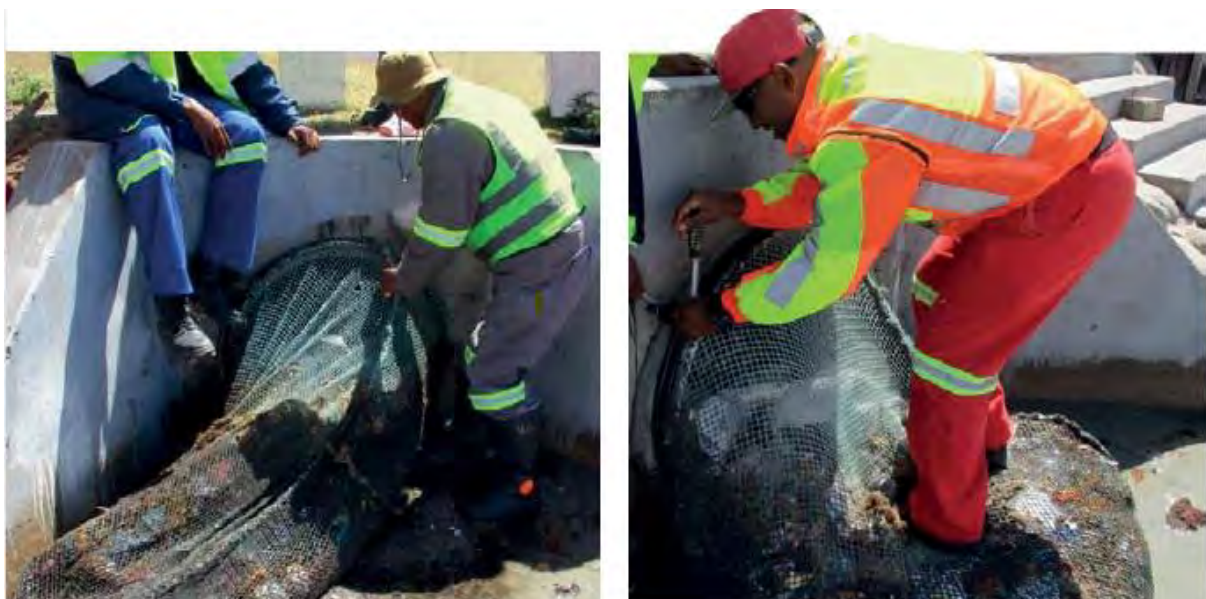
Figure 3-44 A stormwater litter trap installed in Saldanha Bay to prevent litter entering the Bay (Source: SADSTIA annual report 2019).
