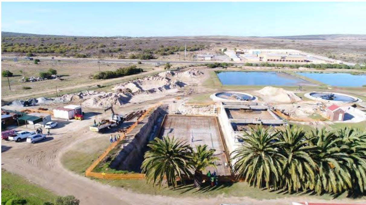
**Figure 3.28** Construction activities for the upgrade of the Langebaan Waste Water Treatment Plant to increase treatment capacity and improve treatment processes (Source: Saldanha Bay Municipality).
