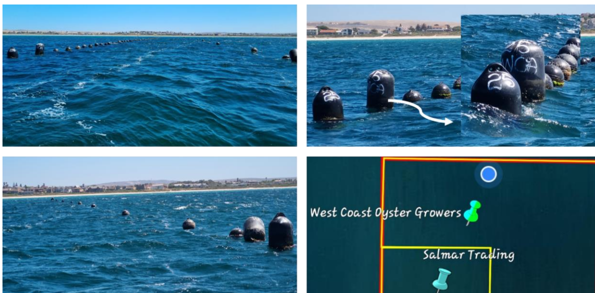
Figure 3.2. All mussel lines at WCOG were observed to be taut, straight, suitably floated (top and bottom left). However, marked with incorrect unique identifiers (top right). Live Google Earth pin of location of compliance photograph in relation to the WCOG SB licence area (yellow boundaries) (bottom right)
