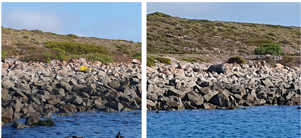
Figure 3.4. Small Bay (Marucs Island causeway) beach inspection.
